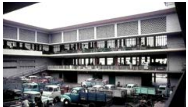
Figure 5. Cobogós at the façades facing the cloister (c.1960s). Luanda, Imagens dos velhos tempos [online].
