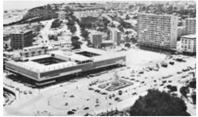
Figure 3. Aerial view of the Kinaxixe Market with Cuca building in 1971. Luanda, Imagens dos velhos tempos [online].
