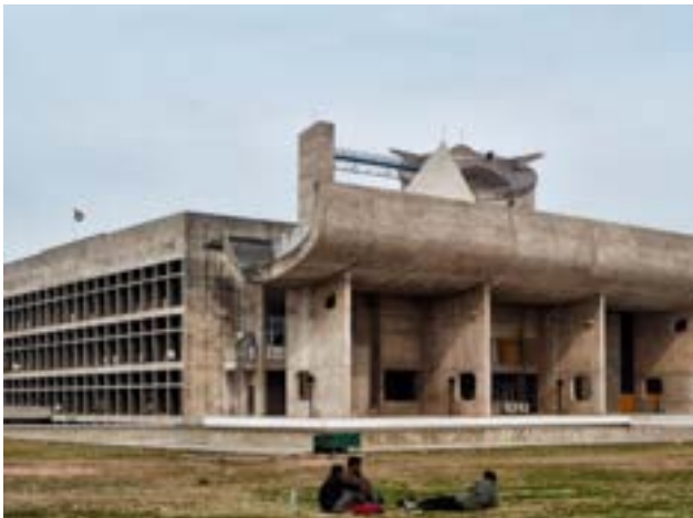
Figure 5. Palace of the Assembly, Chandigarh, Le Corbusier. Cemal Emden, archeyes.com [online].
