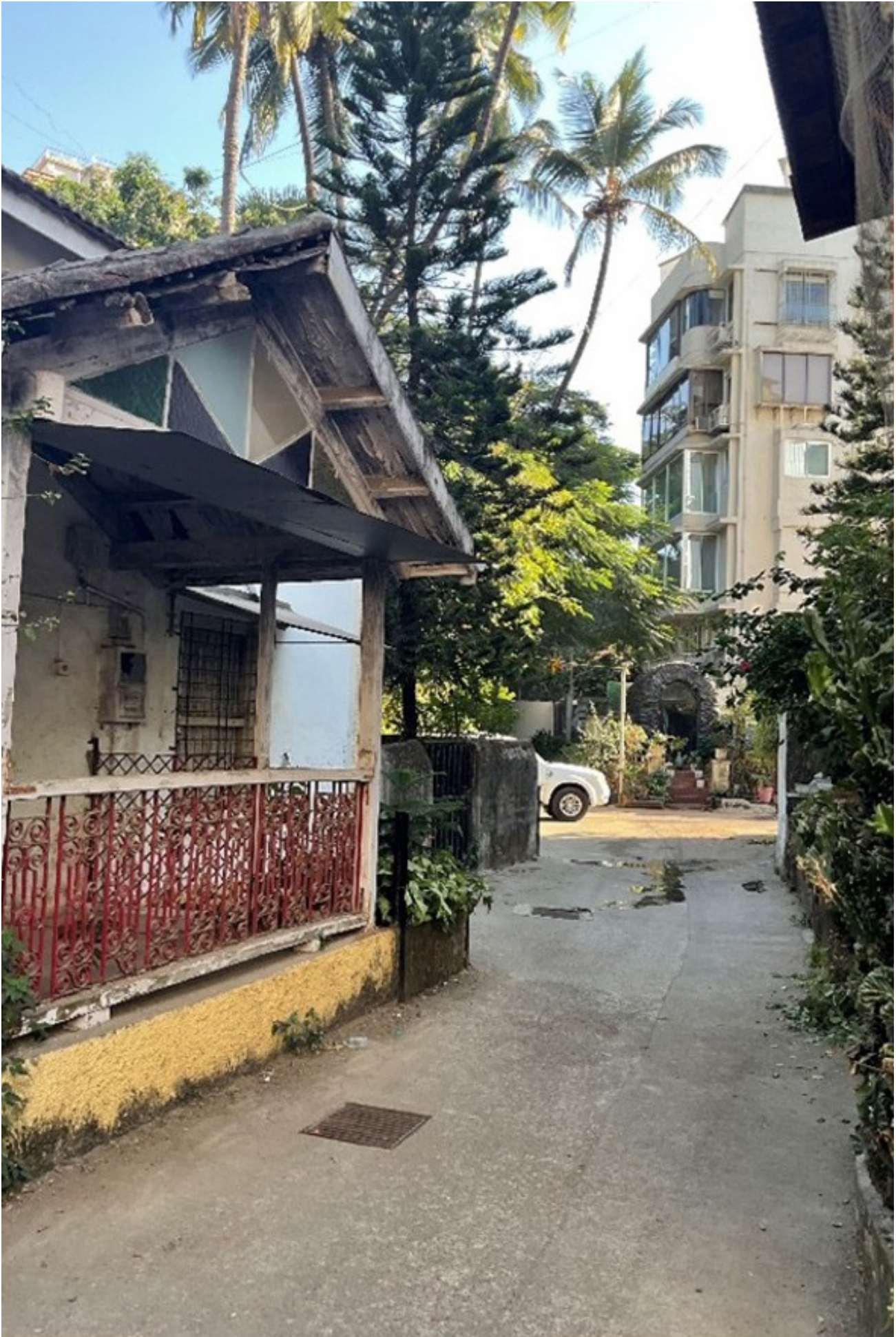
Figure 7. Extensive use of timber in the balcony and beams. Author, 2025.
