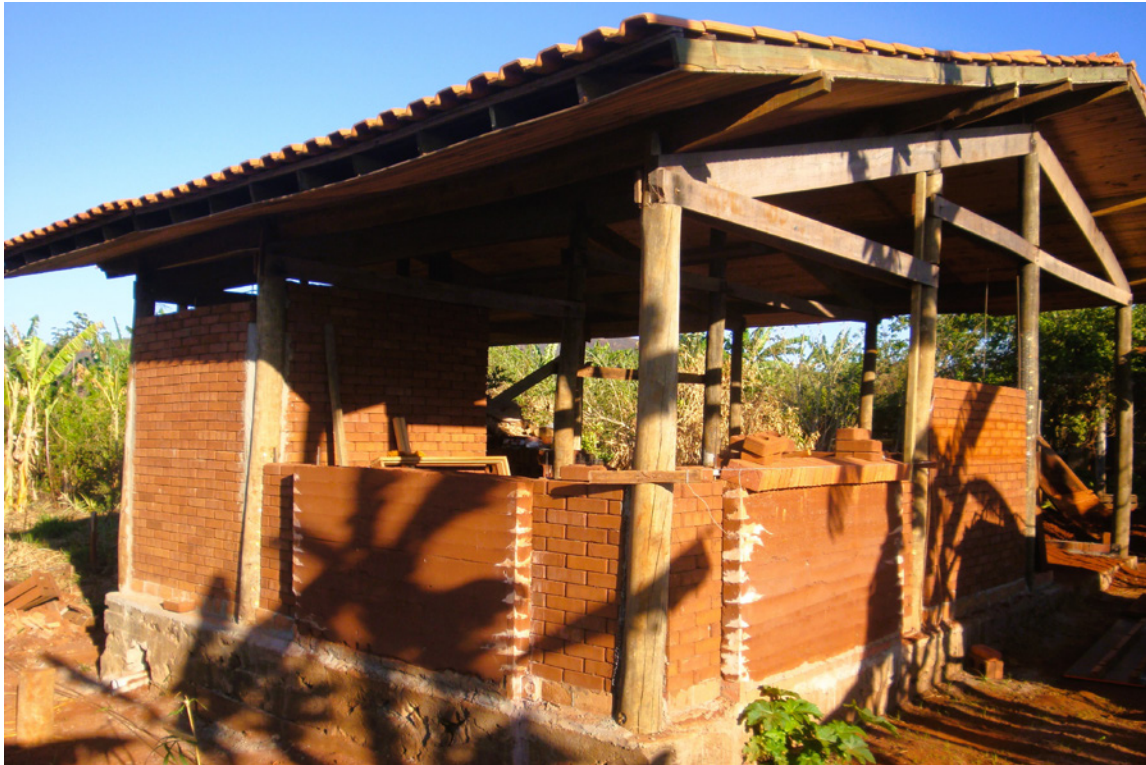
Figure 3. Sepé Tiaraju rural settlement house designed and built by teachers, undergrad students and settlers with mixed low carbon construction techniques (2010). HABIS Archive.
