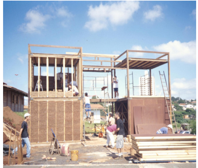
Figure 1. Unit 002 under construction (1997). HABIS Archive.
