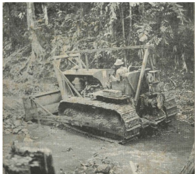
Figure 1. Machinery used during the construction of the City of Golfito. Golfito, a History of the Conquest of the Jungle, n.d. Document provided by the Documentation Centre of the Centre for Historical Research of Central America, University of Costa Rica.
