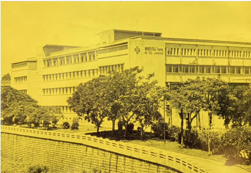
Facade of the Hospital S. Januário, 1974 Back cover image of the Hospital's Inauguration First Centenary Commemorative Edition
