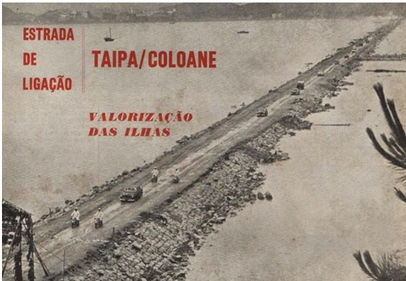
Taipa, Coloane connection road
